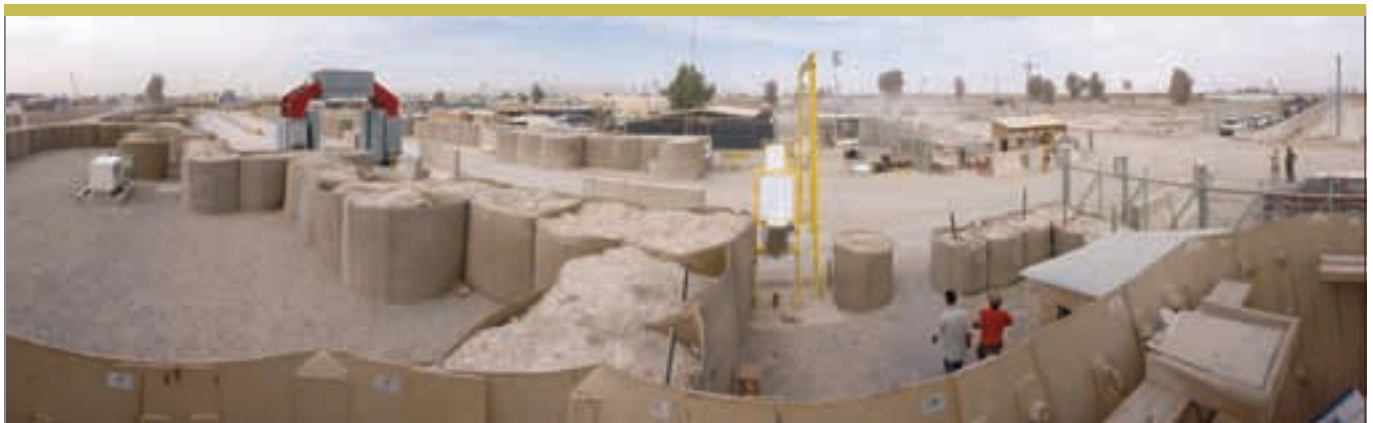
This panoramic picture allows viewing the whole processing area, which includes the scanning area, a waiting area where the vehicle awaits the results of the scan, and a containment area where the vehicle is directed if something suspicious is detected. (NC3A)
