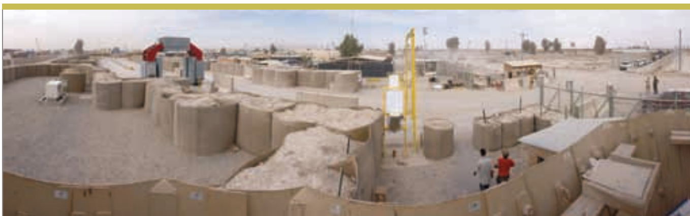
This panoramic picture allows viewing the whole processing area, which includes the scanning area, a waiting area where the vehicle awaits the results of the scan, and a containment area where the vehicle is directed if something suspicious is detected. (NC3A)
